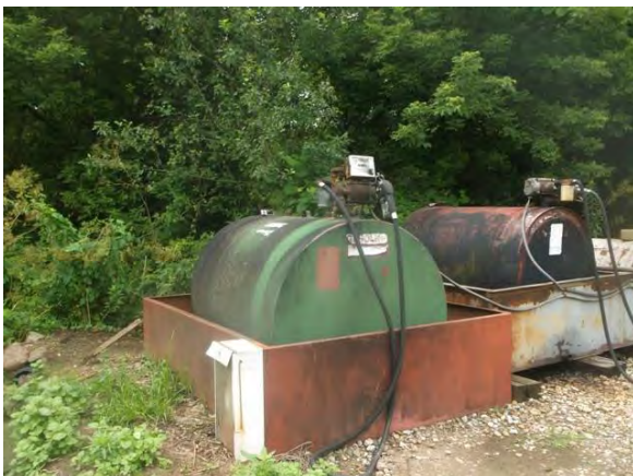
Photo #11: One 500-gallon gasoline AST and one 500-gallon diesel AST located in the southeastern portion of the maintenance area.
