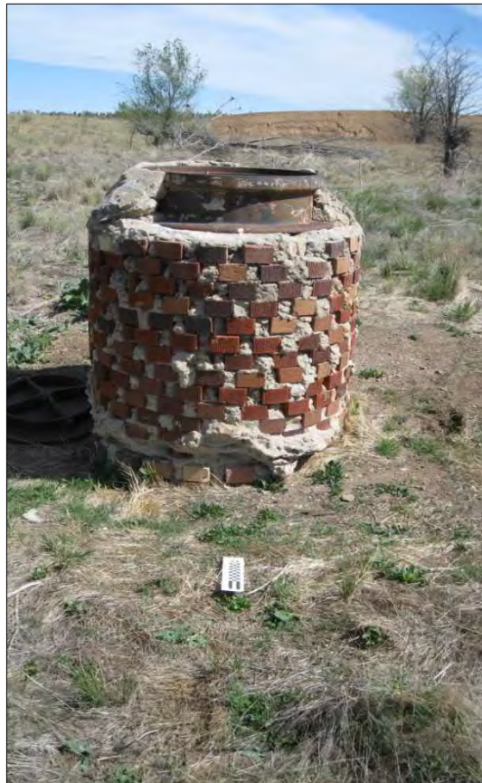
Figure 7. HRA-FL1, raised brick and mortar manhole cover.
