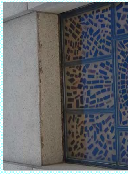
Photo: F—Moisture staining at window header on exterior
