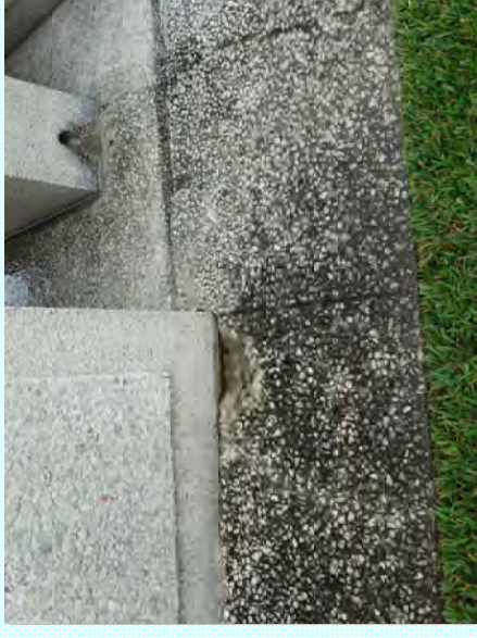
Photo: N —Large divots at base of panels and flatwork
