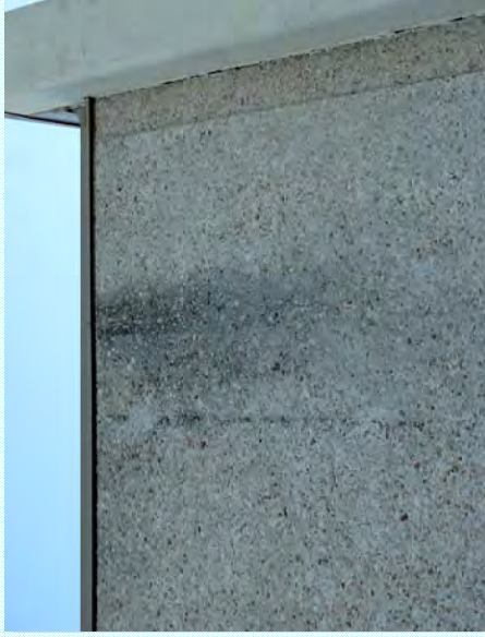
Photo: I—Moisture staining, typical
