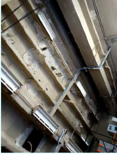
Photo: A—Coating in the garage at ceiling is peeling off
