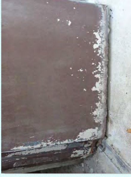
Photo: KK—Hollow metal door at the base of the tower is rusted through
