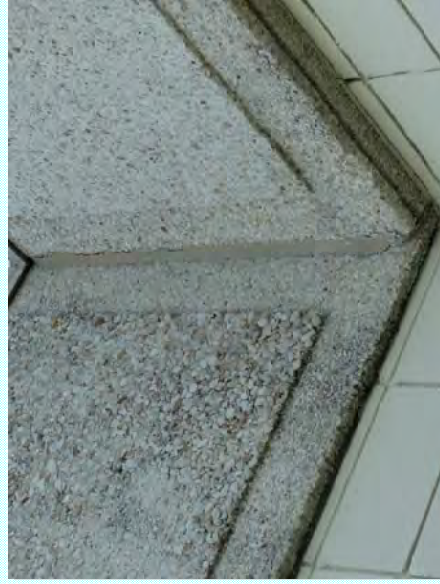
Photo: G—Sealant joint is unsound
