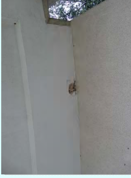
Photo: Y—Severe spalling at decking, exposed reinforcing steel
