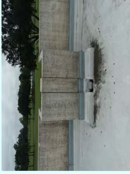
Photo: R—Horizontal cracking at inside of upper panel
