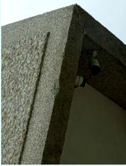
Photo: A—Chipped edge at bottom of floating panel
