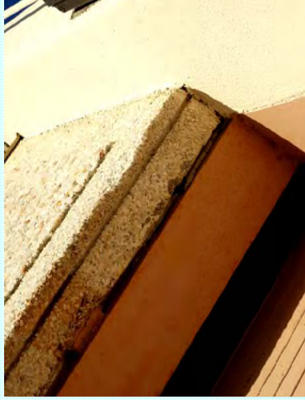
Photo: E—Underside of floating panel is damaged and missing sealant
