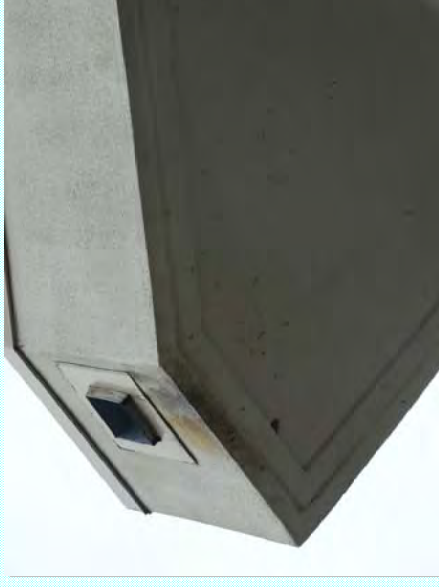
Photo: EE—Staining at podium canopy scupper
