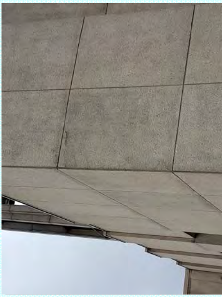
Photo: E—Horizontal cracking at upper corner of panel
