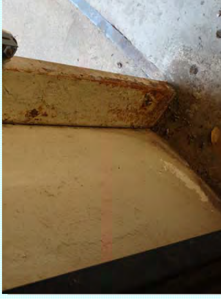
Photo: D—Metal door frame is beginning to rust at the base
