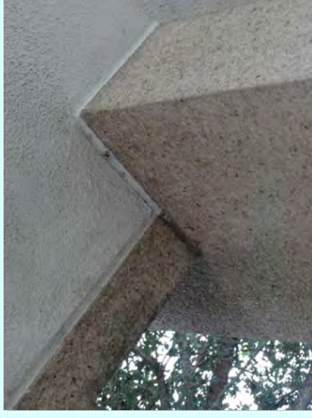
Photo: W—Visual observation of water seeping through deck
