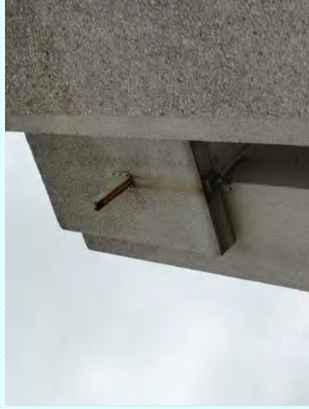
Photo: K—Rust staining from flag pole mounts
