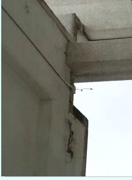
Photo: L—Exposed speaker conduit and wires
