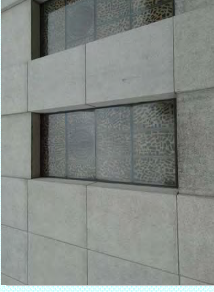
Photo: D—Existing storm panels show signs of movement
