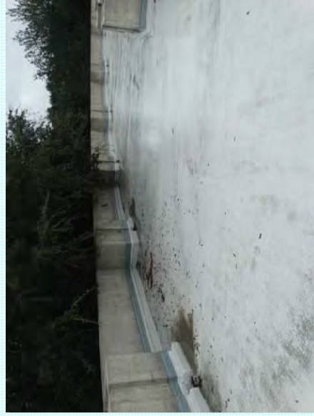
Photo: S & T—Tree overgrowth onto upper deck and ponding
