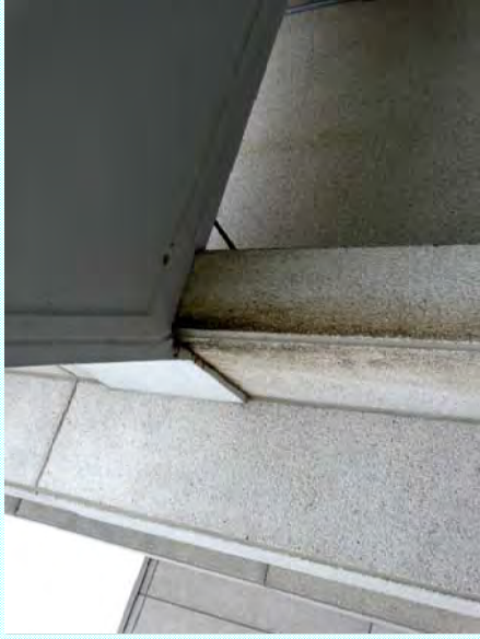
Photo: DD—Biological growth and staining at podium canopy
