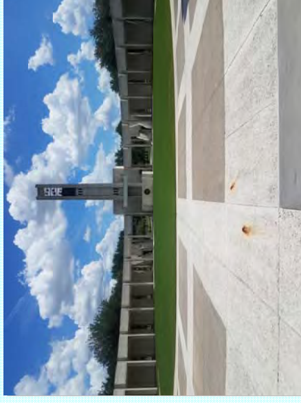
Photo: J—Rust staining on site flatwork at east plaza
