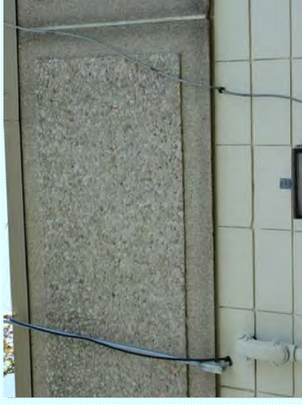
Photo: F—Several penetrations are not sealed properly
