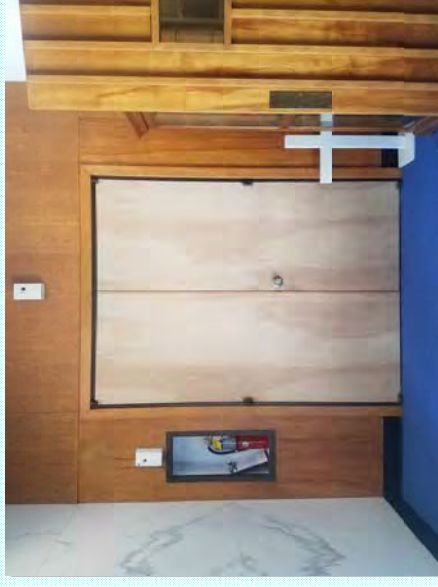
Photo: M—Wood doors at vestibule are unfinished
