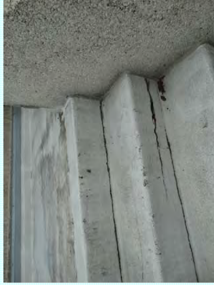
Photo: BB—Horizontal cracking at stair riser
