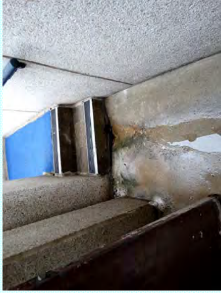
Photo: HH—Water ponding, biological growth and failing sealants
