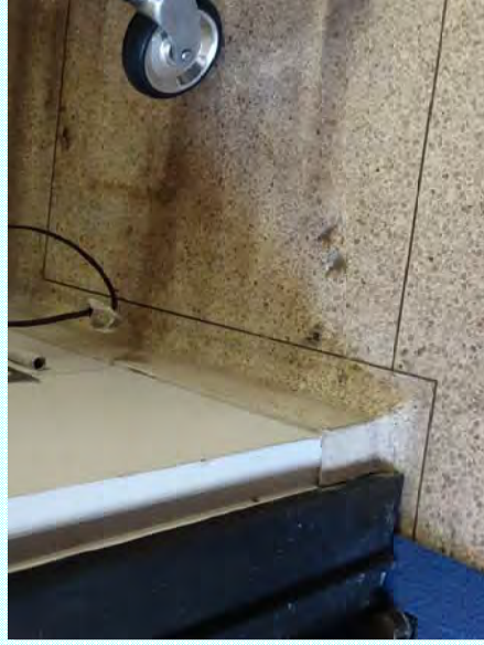
Photo: R—Two areas of minor terrazzo floor damage
