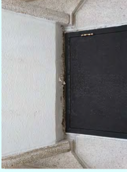
Photo: U—Biological growth and finish spalling at header of door
