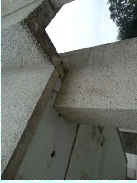
Photo: AA—Severe cracking at underside of upper panels
