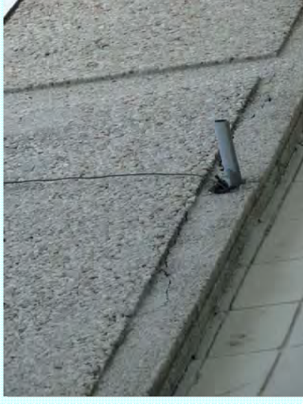
Photo: J—Cracking at penetration on South Elevation
