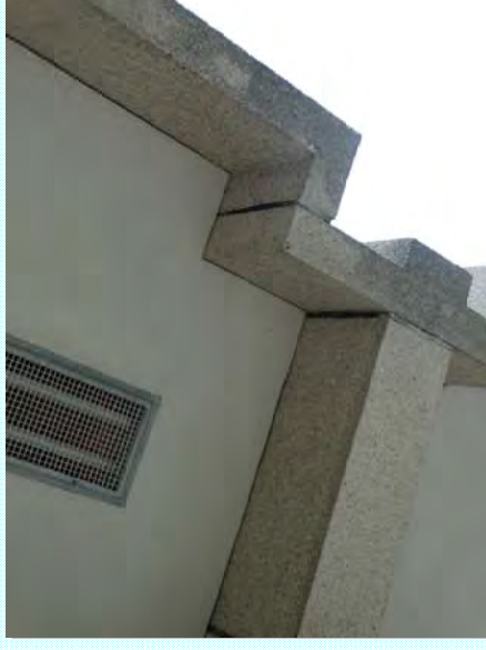
Photo: B—Consistent staining at the underside of floating panels
