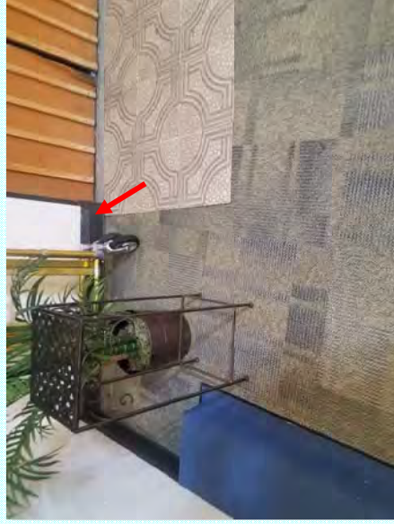
Photo: N—There is a black rubber base over the original marble base
