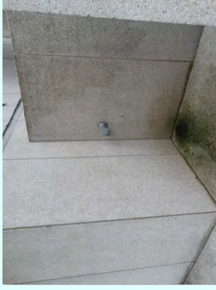
Photo: II—Biological growth at speaker canopy drainage to site
