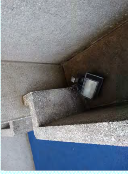
Photo: GG—Failing sealant, water ponding and staining at light wells
