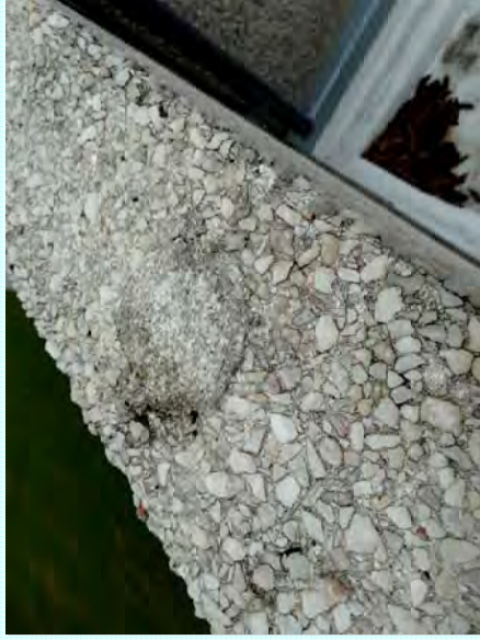
Photo: Q—Biological growth on previous patchwork at top of panel
