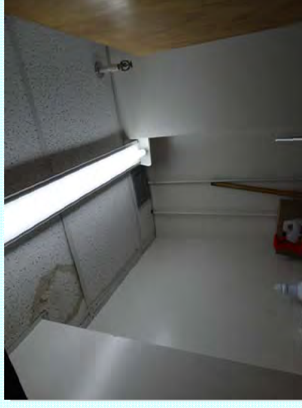
Photo: O—Acoustic ceiling tiles in janitor contain moisture damage
