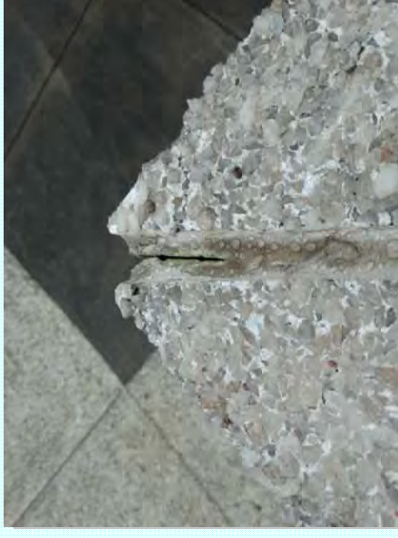
Photo: CC—Sealant joints separation and deterioration
