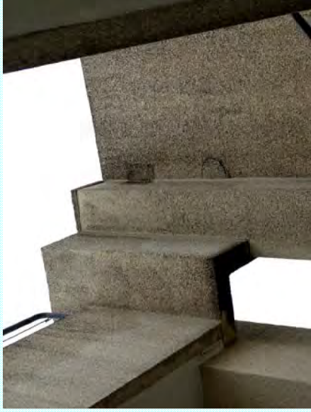
Photo: M —Cracking and spalling at embedded steel anchors
