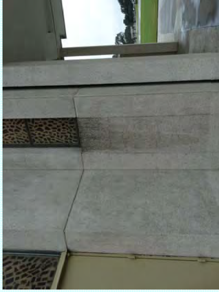
Photo: C—Moisture staining at window sills, typical
