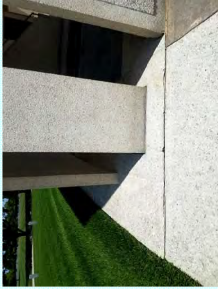
Photo: I—Failing sealant at site concrete flatwork
