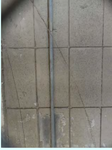
Photo: B—Coating in garage at wall is spalling off
