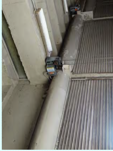
Photo: C—Coating in the garage at the overhead door is peeling off
