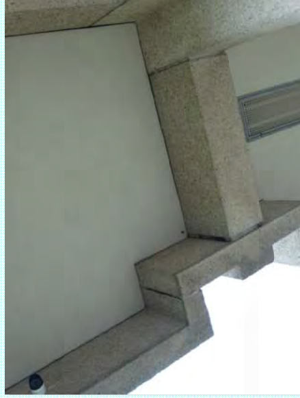
Photo: C—Consistent staining and biological growth on concrete panel joints
