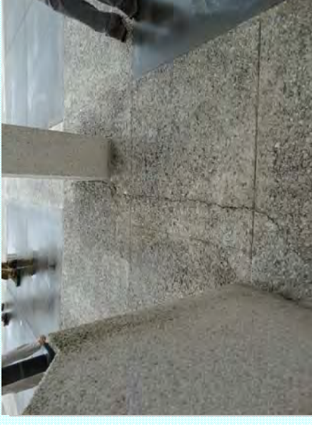
Photo: P —Large divots and cracks at base of column and flatwork
