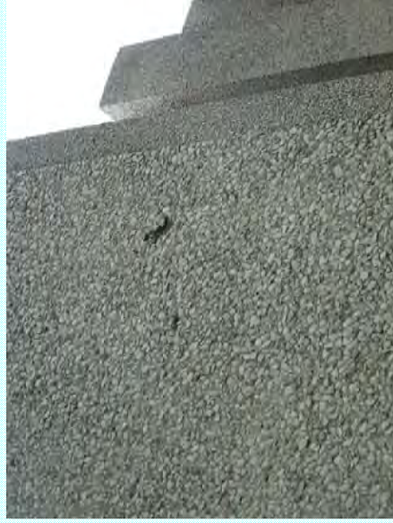
Photo: X—Divots at concrete panel
