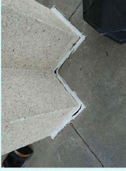
Photo: D—Deteriorated sealant at flatwork along building footprint
