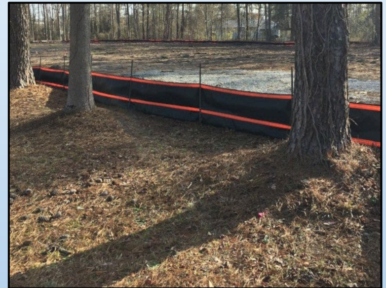
Best management practices for protecting water quality from sediment in stormwater runoff will be implemented during construction.
