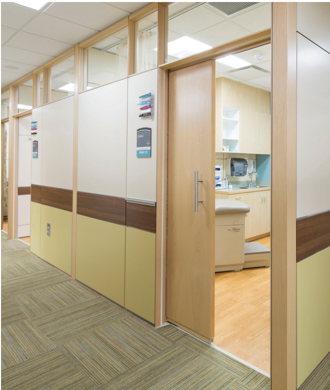
Figure 8.4 Panelized structure as interior fit-out, DIRTT
