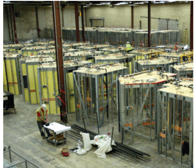
Figure 8.1 Prefabricated toilet room components, Skanska
