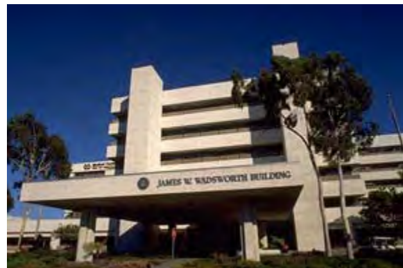
VA Medical Center West Los Angeles, CA, 1976 (not VAHBS, used interstitial space)
