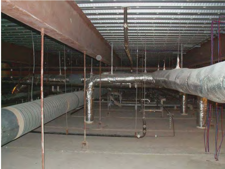
Photo A-9 Interstitial Service Zone Showing remodel work
