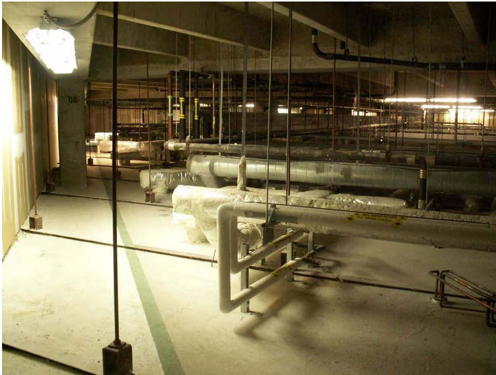
Photo C-4 Interstitial Service Zone
