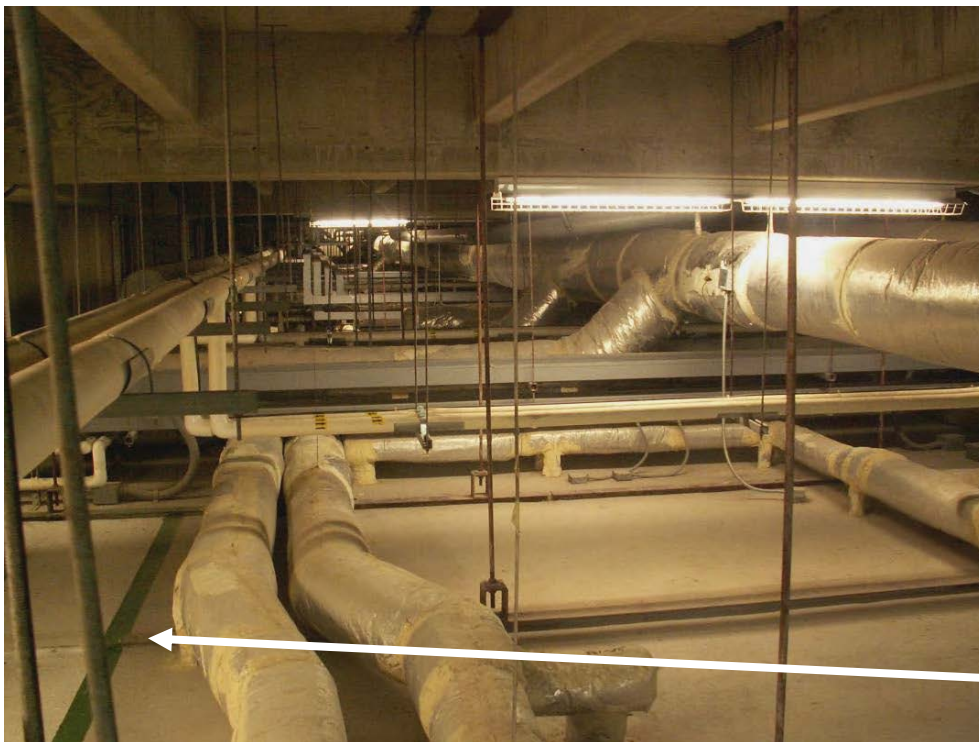
Photo C-8 Interstitial Service Zone
