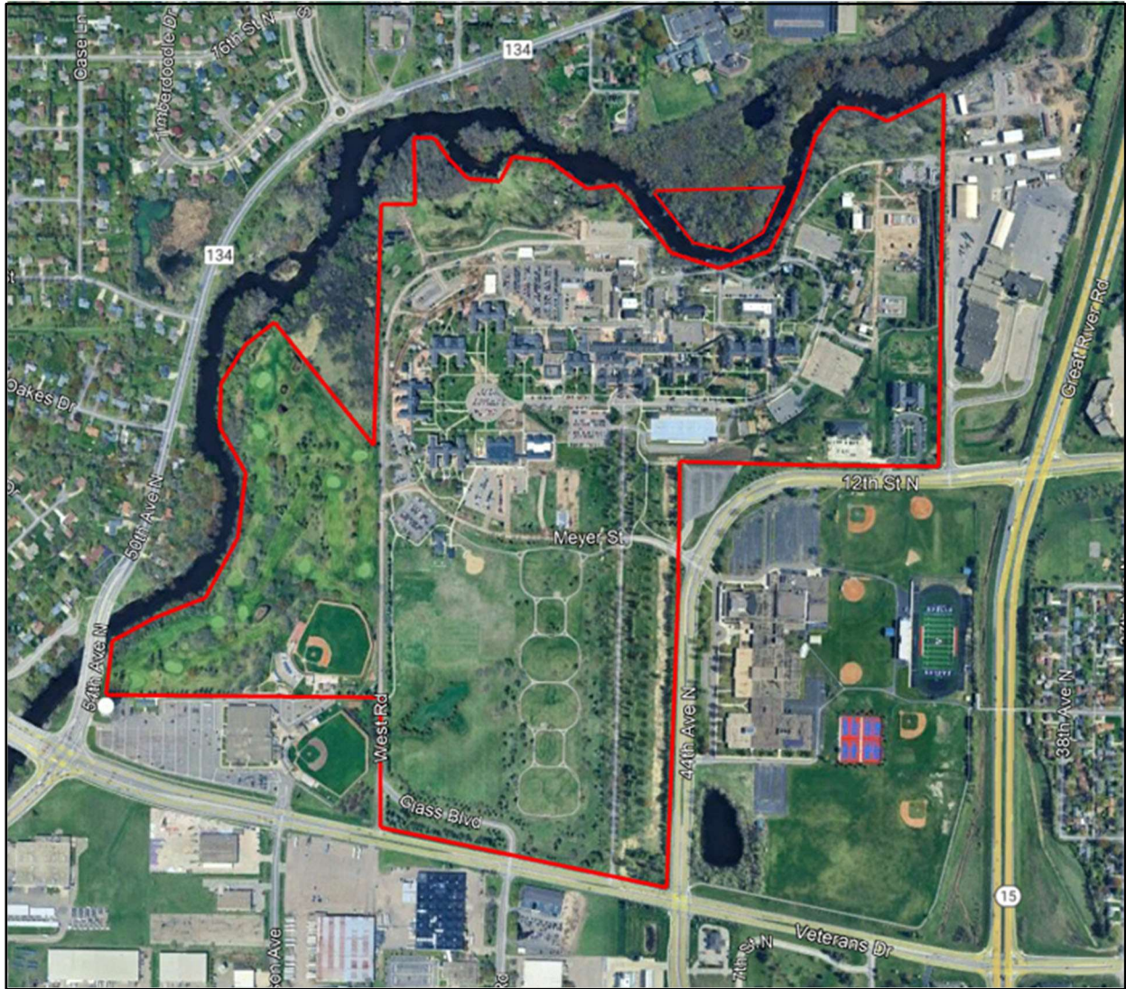
Figure 3: Aerial Photograph of St. Cloud VAMC Campus
