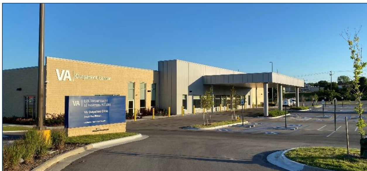
Figure 3 - VA Outpatient Clinic in south Des Moines, Iowa. This clinic was a former Toys R Us and modified (Build-Out).
