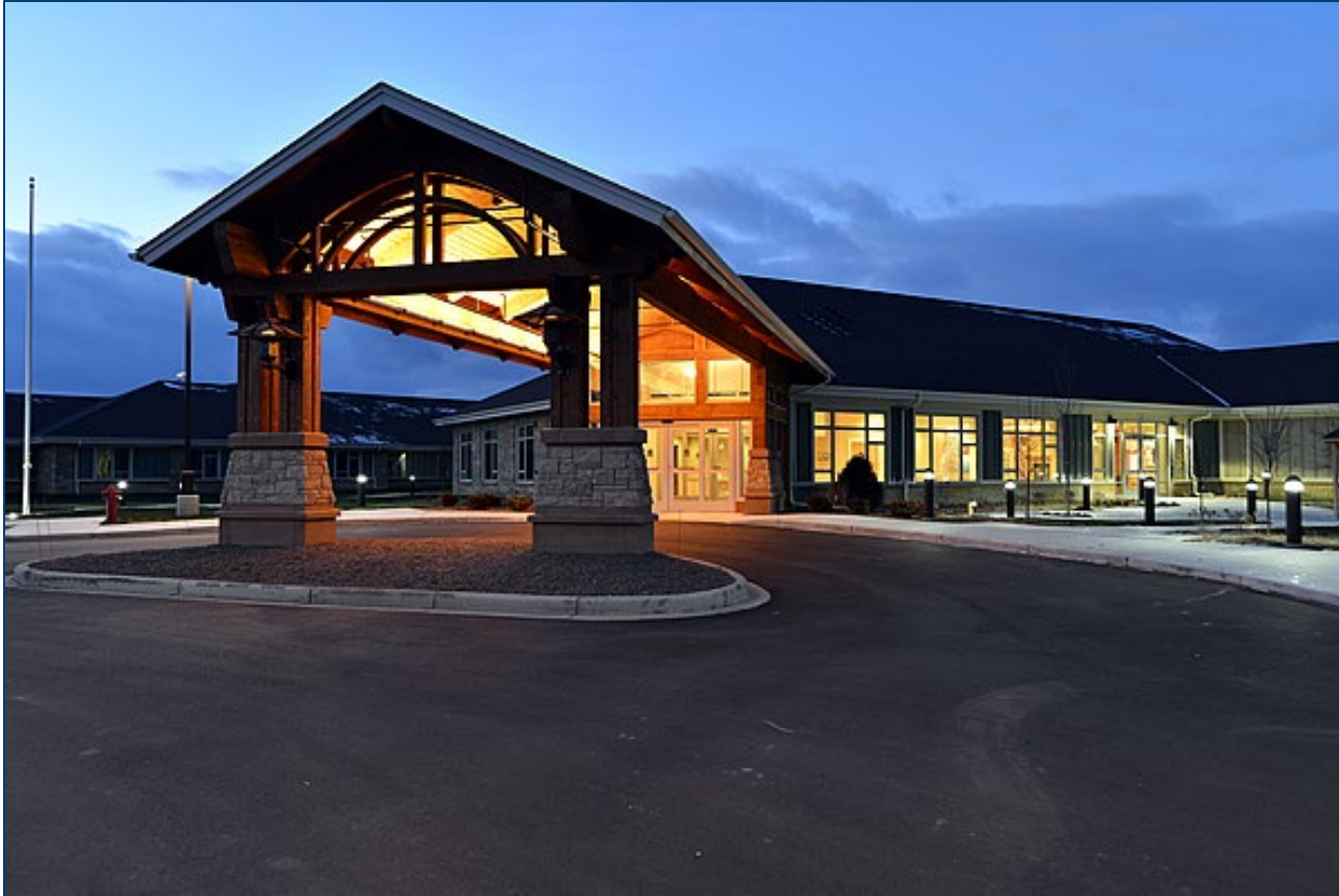
Wisconsin Veterans Home at Chippewa Falls
